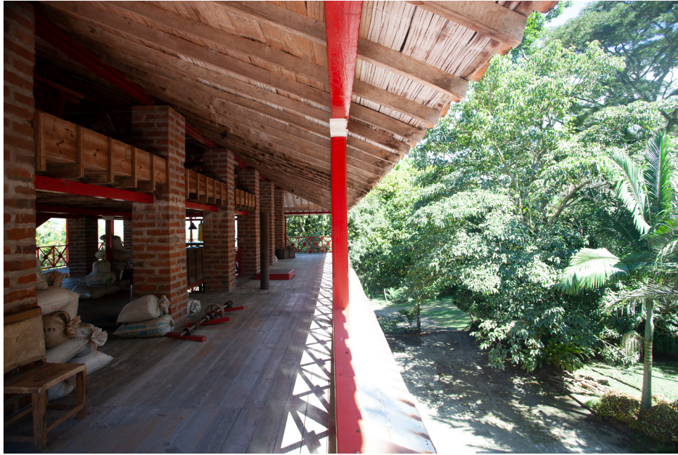
Fig. 12. Eave and corridor at vernacular coffee wet mill from early XX century, Tarso, Antioquia, Colombia
