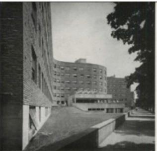
Available building materials often suggest different forms of expression. Aalto's student apartments at M.I.T. curved up in the shape of a whiplash curve partly because concrete and brick permit—and even suggest—such forms. Wurster's office building in San Francisco, Calif., made a virtue of straight lines (and emphasized their straightness with long horizontal lines) because wood is essentially a straight material. Yet, in spite of the two buildings have much in common.
