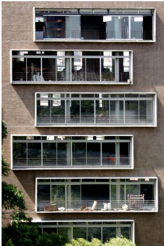
Fig. 13. Perimeter corridor in Calle 10b Housing, Medellín. Camilo Restrepo Ochoa and J.Paul Restrepo.
